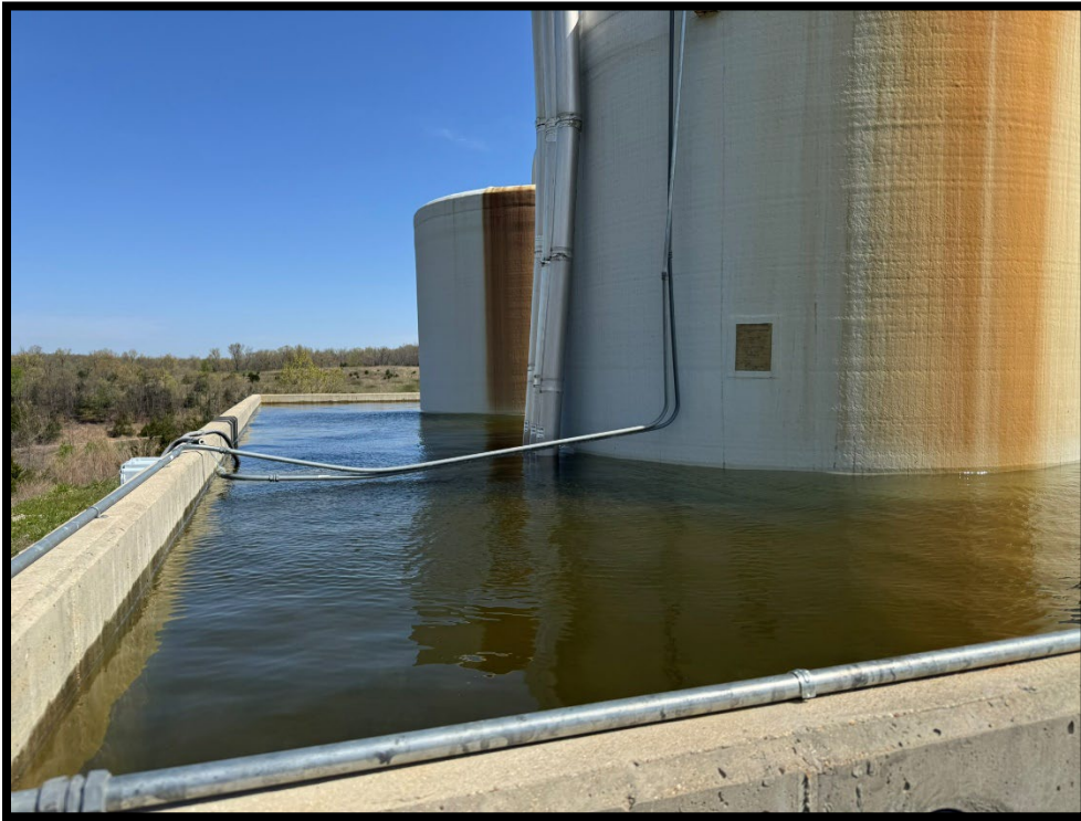
Photograph 3: View of leachate tank containment near capacity and staining on sides of tanks.
