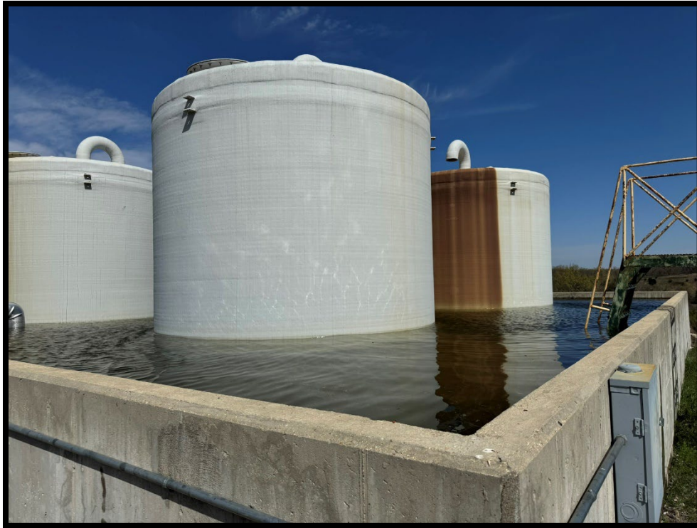
Photograph 5: View of leachate tank containment near capacity and staining on side of tank.
