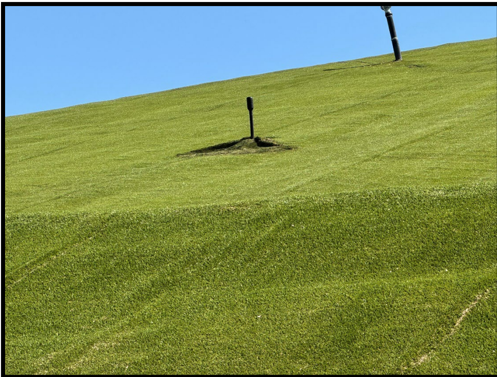
Photograph 8: View of damaged turf around PRV on north side of Area 1-2.
