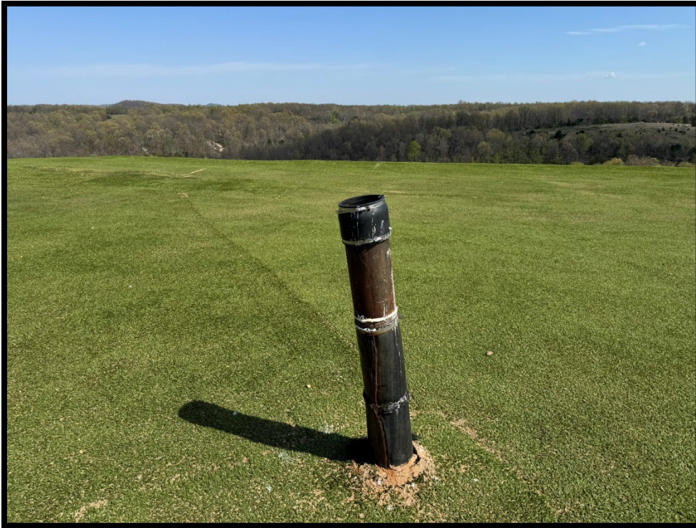
Photograph 7: View of detached turbine vent on north side of Area 1-2.
