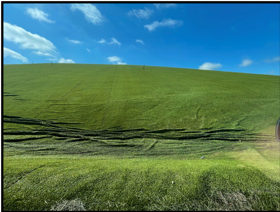
Photograph 6: View of rills in closure turf on the north side of Area 1-2.
