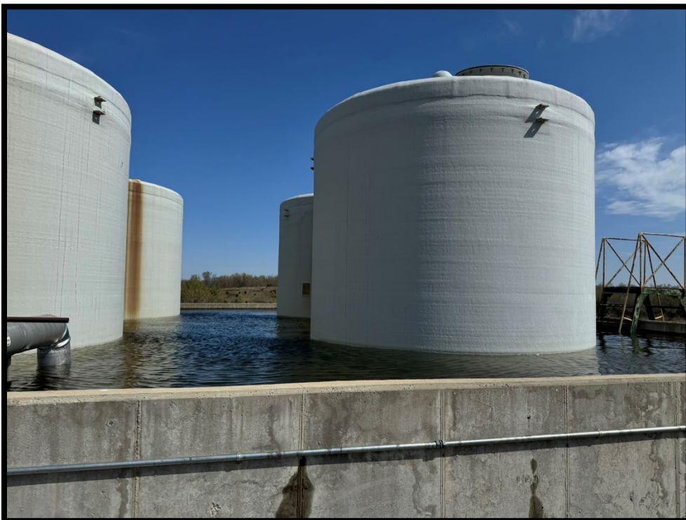
Photograph 4: View of leachate tank containment near capacity.
